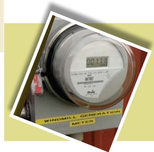
Sensing's meter shows that he is using less electricity because of his wind turbine.
