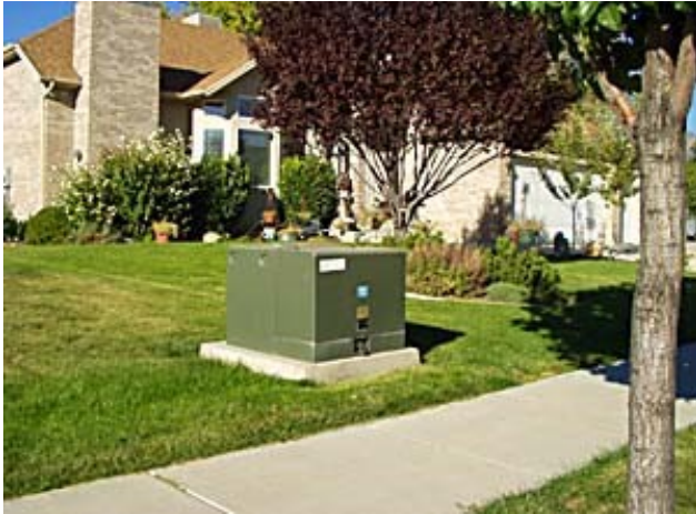
Figure 1A: Pad-mounted Equipment (Underground System)
