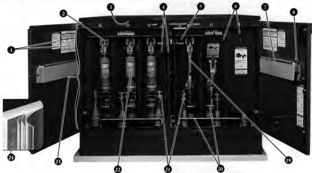
Figure 9. Fuse-side view of a Model PMH-9 with SML-20 Power Fuses in the right-hand compartment and Fault Fiter Electronic Power Fuses in the left-hand compartment. (This nonstandard combination of fuses is shown for comparison only.)
