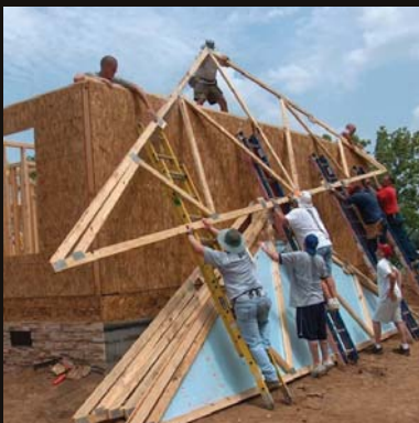
NES employees helped build seven new homes with Habitat for Humanity.
