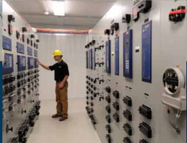
After: The NES system downtown is now almost entirely below ground.
